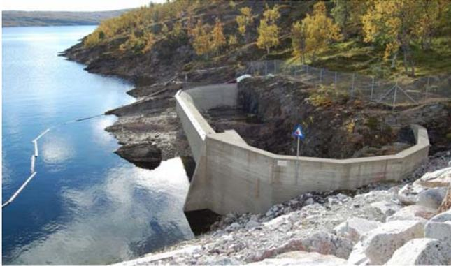
Figure 1. Photograph of the spillway structure at the Innerdalen Dam (Vingerhagen, 2011)
